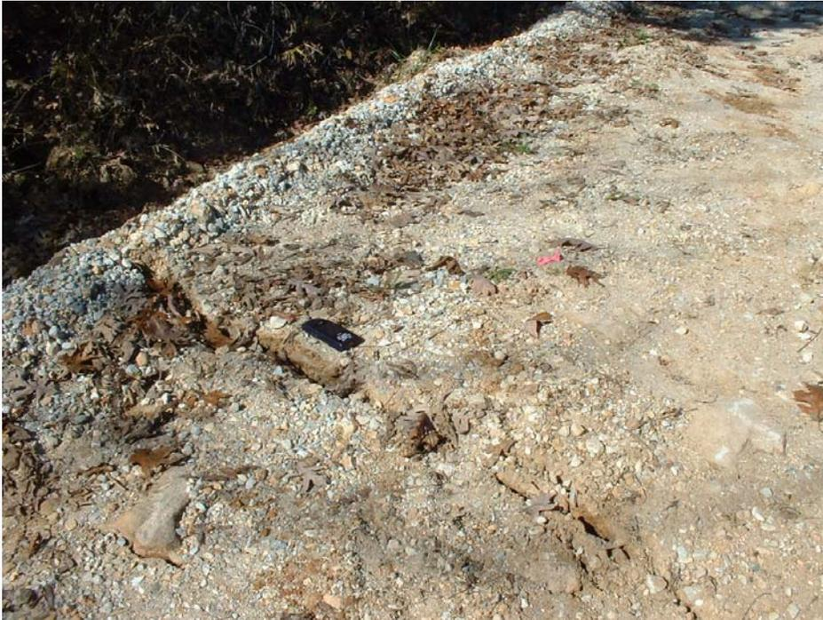
“Hump” and crack in road near Pin #3 on Blackjack Lane. Tensional crack trends N80°E and is down dropped ~1 inch to the south. Latitude: 36.18156, Longitude: -93.19998.
