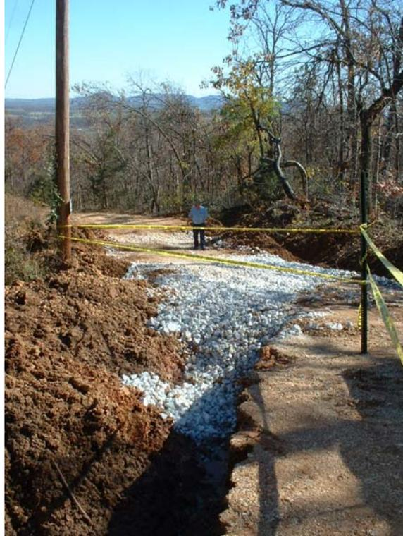
View looking east down slope from west scarp line on Ridge Court Road. Note hummocky nature of road below scarp due to colluvium creep.
