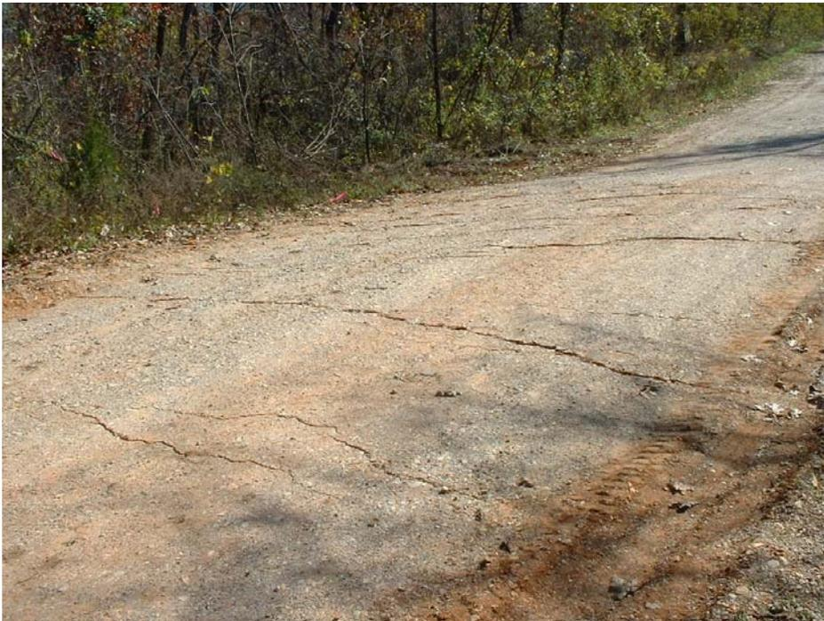
Set of 6 sub-parallel tension cracks trending N130°W in Blackjack Lane. Latitude: 36.18256, Longitude: -93.19981.
