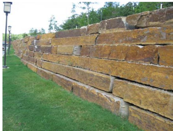
Figure 8. Rock wall made of Arkansas stone.
