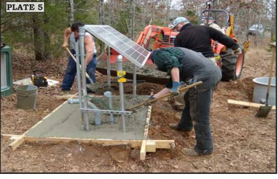
Pouring a 3 inch concrete pad for above-ground equipment enclosure
