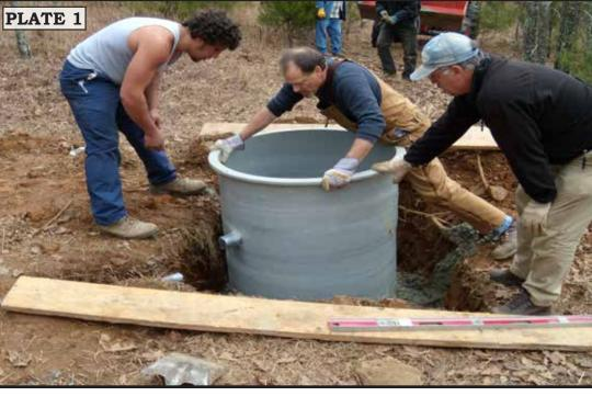
Placing a 3x3.5 ft. cylindrical, fiberglass vault 3 ft. below-ground
