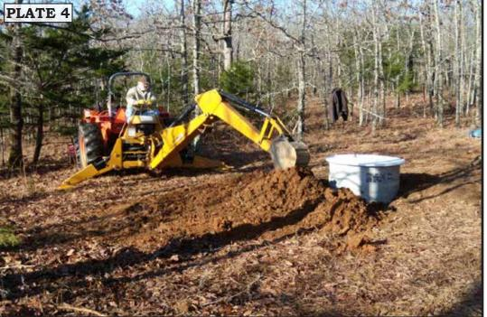
Backfilling around fiberglass vault
