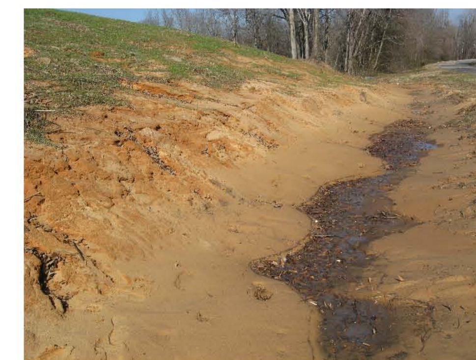
Terrace deposits exposed along Highway 105 south of Atkins.
