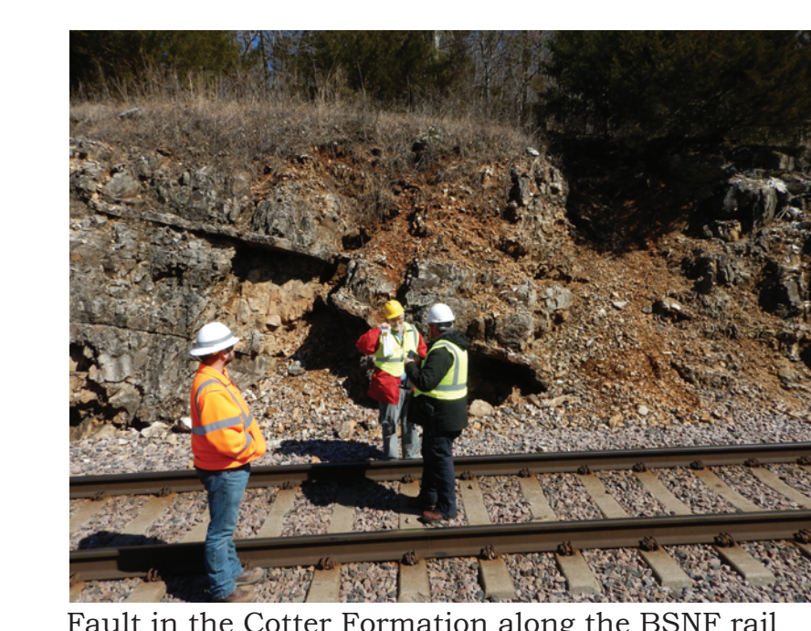
Fault in the Cotter Formation along the BNSF rail line north of Horseshoe Bend.
