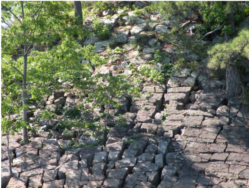
Figure 13. Joint system in the Blakely Sandstone at Checkerboard Rock.
