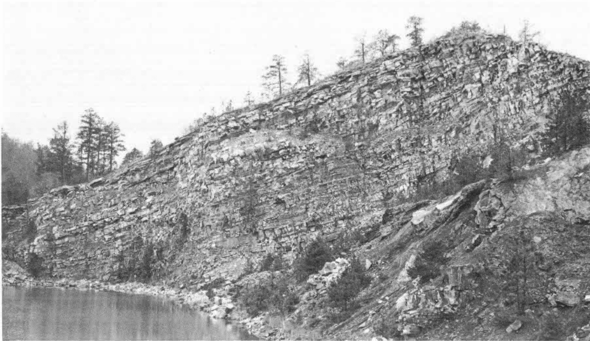
Figure 16 - Stop 7. Quartzitic sandstone of the upper Jackfork Sandstone overlying a faulted olistolithic zone in the black shale of the middle Jackfork Sandstone. This exposure is in the abandoned West Fulk Mountain quarry at the Pinnacle Mountain State Park Visitor Center.
