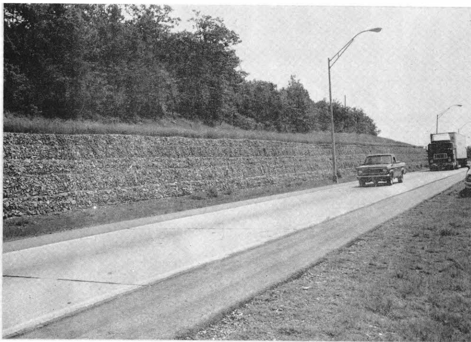
Figure 6 A. -- Gabion wall at exit 10 on I-540 in Fort Smith.
