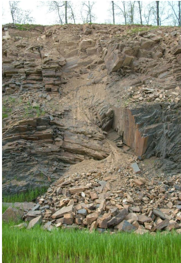
Figure 7. Failure along persistent structural fracture planes: Atoka Formation (sandstone facies) at Interchange #124 on I-40 approximately two miles west of Conway. Strata dip “into” the outcrop. Joint planes dip “out” of the outcrop.
