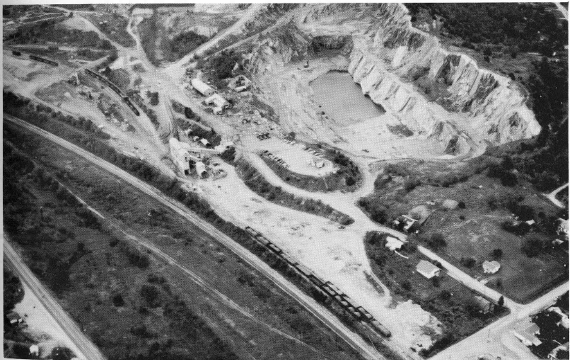
Fig 5.-- Quarry of Southwest Stone Company, Stringtown, Oklahoma. Aerial view northeast. (Photo courtesy Magnolia Petroleum Company)
