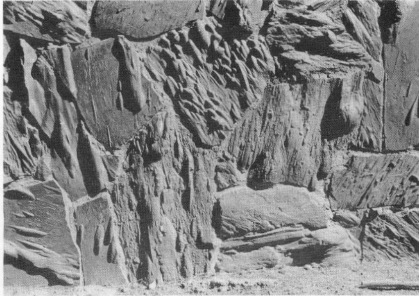
Fig. 26.-- Flute casts, flow casts, groove casts, and load casts characteristic of under surfaces of sandstones of Wildhorse Mountain formation. Widely used as a building stone in the Ouachitas. The Mike Emery dwelling, Kosoma, Oklahoma. (Photograph by L. M. Cline)
