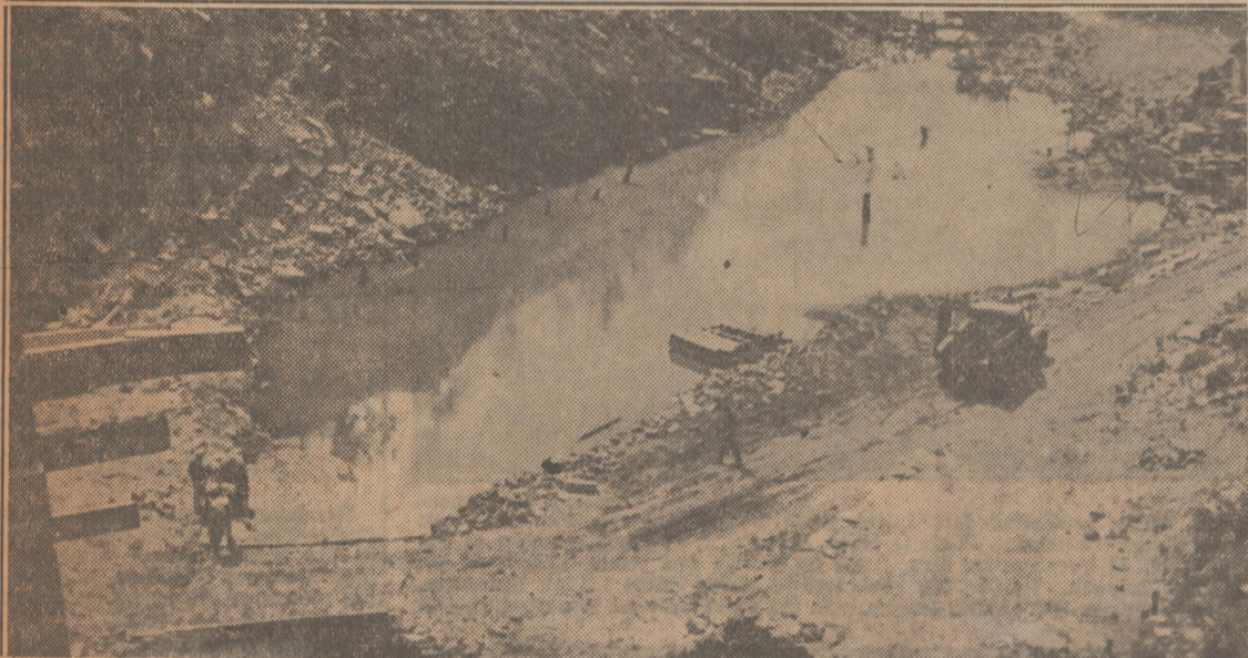
Top, the stone and masonry dam at Spring Creek, near Bellville, a part of the Mount Magazine recreation project, which was finished the past week, and the water gate closed to start the lake. Center, the first of the spring water backing up behind the dam; in other words, the lake is being born here. Lower, the iron gate that impounds the water; it can be raised as an emergency valve if the lake level approaches the top of the dam.
